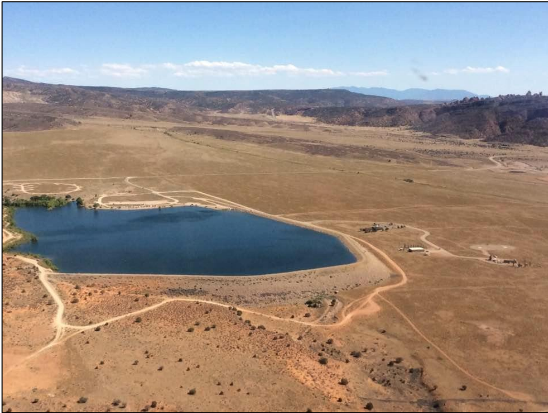
Aerial view of Moab Interagency Fire Center August 2017
